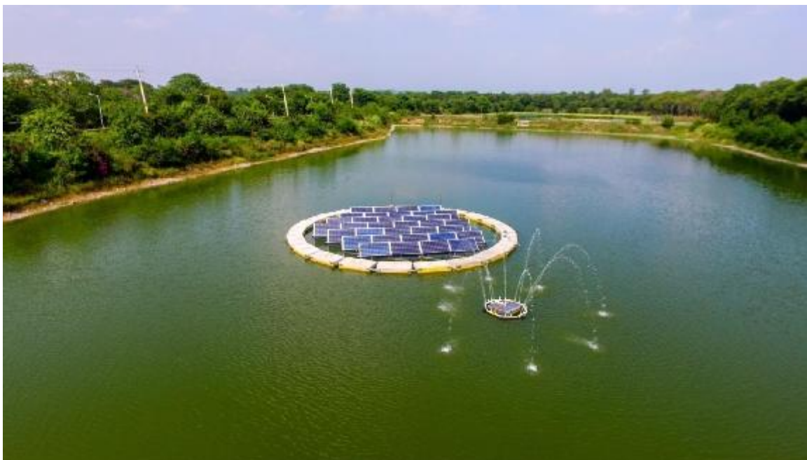
Fig.2:- Photovoltaic Floating Solar Plant
