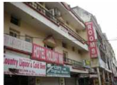
COMMERCIAL ACTIVITY SPREAD ACROSS FLOORS
