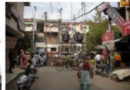
HANGING WIRES-TRANSFORMERS ON MAIN STREETS
