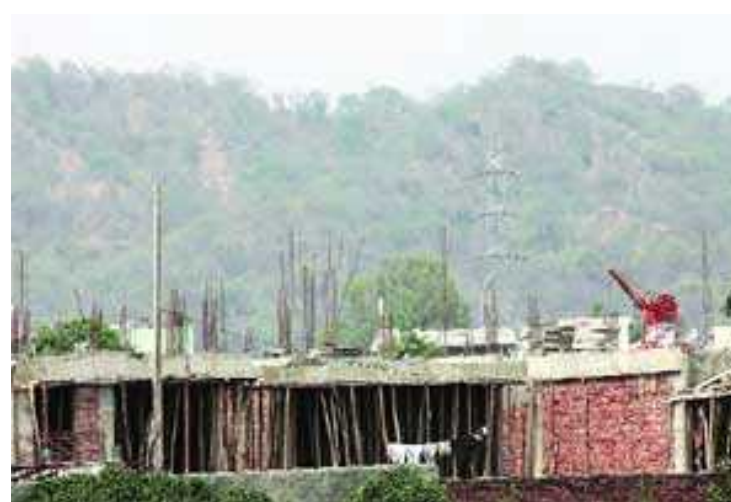
Construction of School and village Kaimbwala
