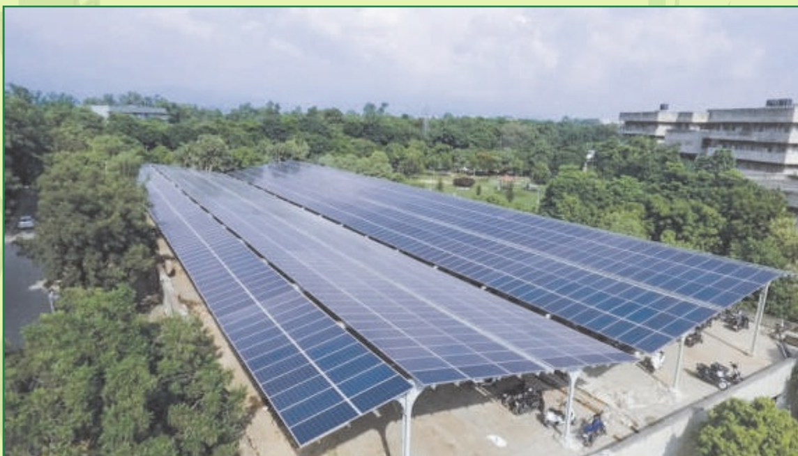
450 kWp Rooftop Solar Photovoltaic Power Plant at Two Wheeler Parking area, Govt. Medical College & Hospital, Sec.32, Chandigarh
