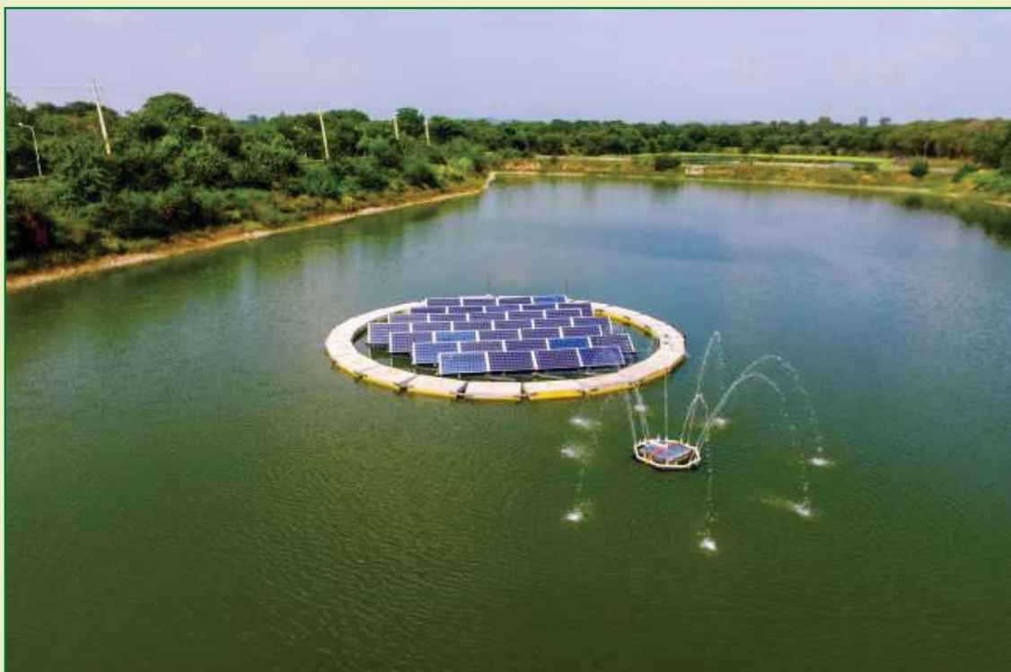
10 kWp floating Solar Photovoltaic Power Plant with fountain at Dhanas Lake, Chandigarh
