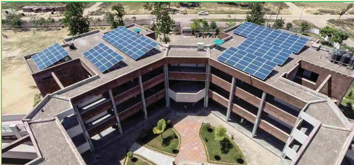
40kWp Grid tied Rooftop Solar Photovoltaic Power Plant at Govt. High School Smart Sector 53, Chandigarh.
