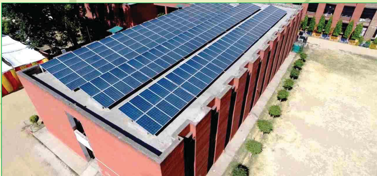
60kWp Grid tied Rooftop Solar Photovoltaic Power Plant at Govt. Sr. Sec. School Dhanas, Chandigarh.
