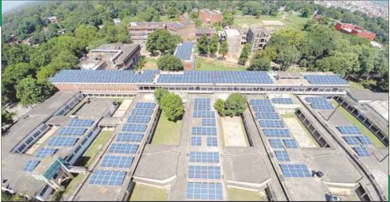
1000 kWp Rooftop Solar Plant installed at Punjab Engineering College, Sector-12, Chandigarh.
