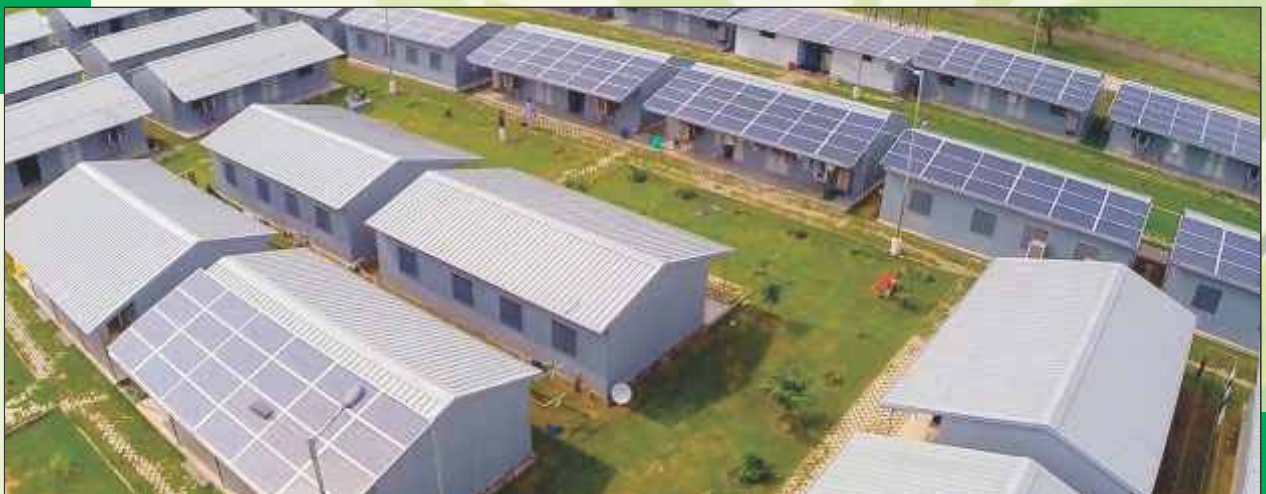
200 kWp Grid tied Rooftop Solar Photovoltaic Power Plant on 22 Huts (Porta cabins) at IRB Complex, Sarangpur.
